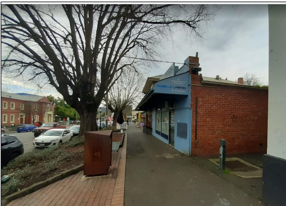
Figure 2 Frontage facing East
