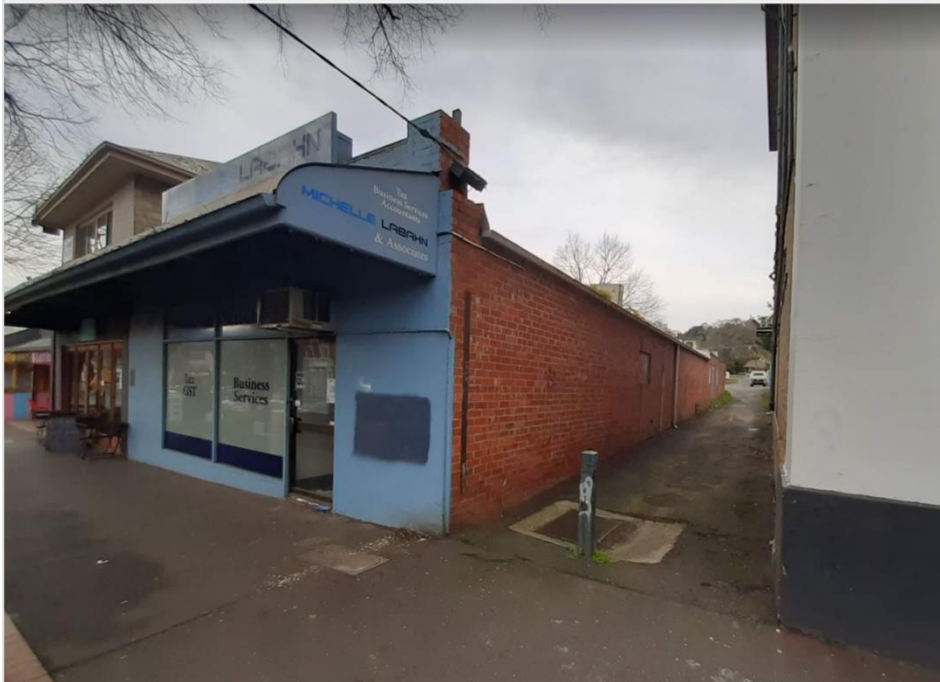
Figure 1 Site Building Frontage
