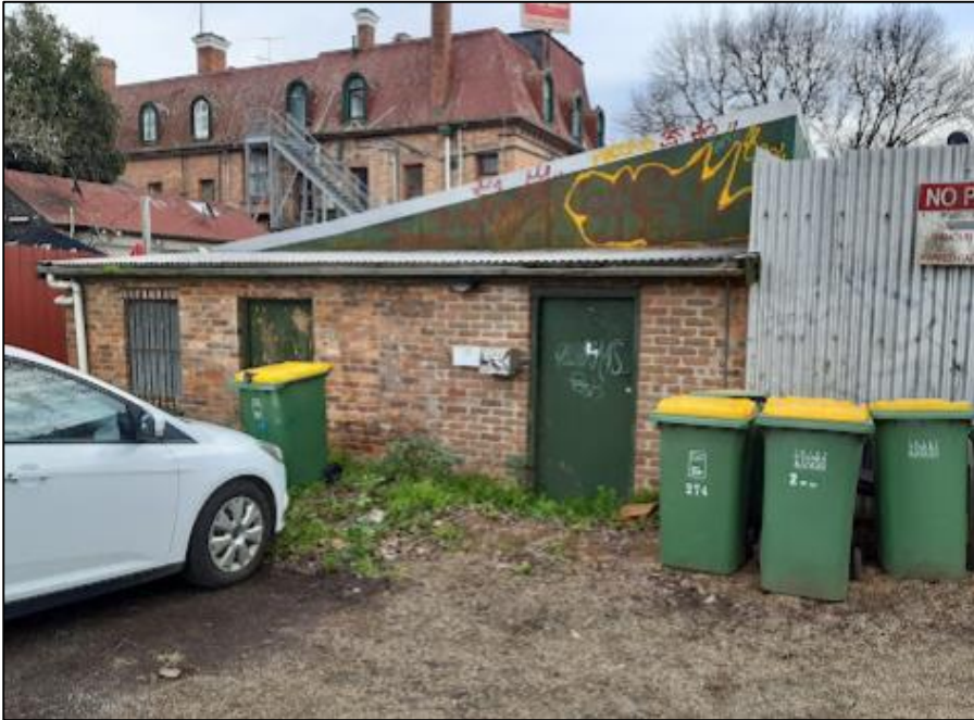
Figure 6 Common parking area facing North (closer)
