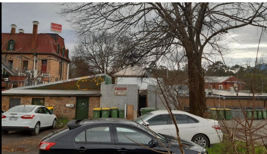
Figure 5 Common parking area facing North
