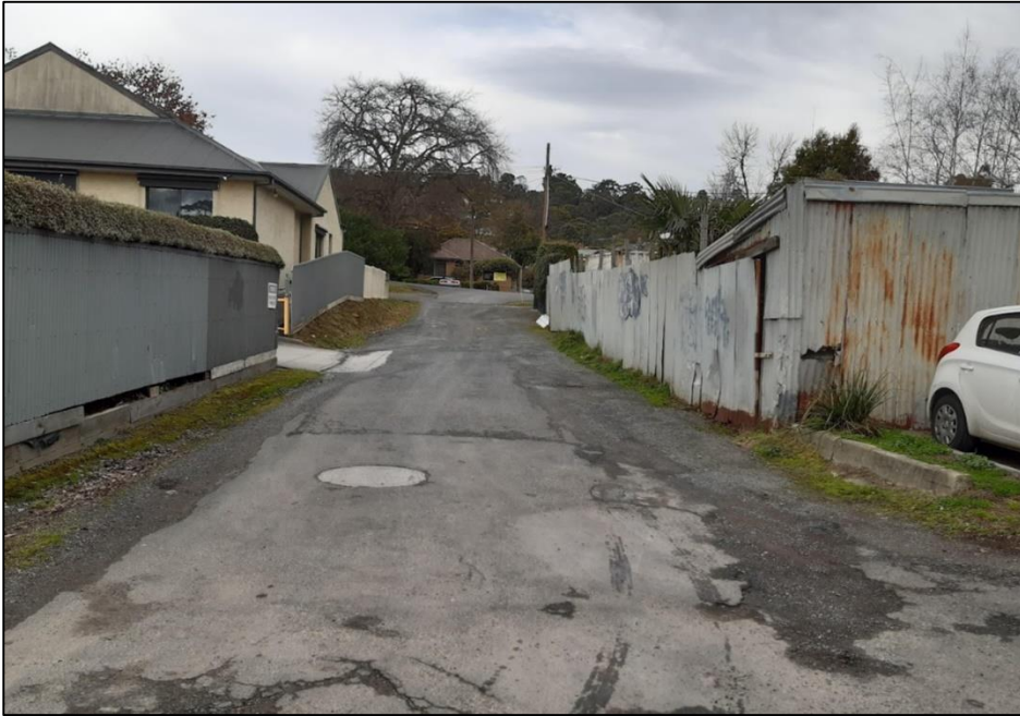
Figure 8 Council Road from Symon Street – lending to carpark- south facing
